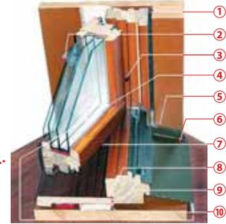
1. Vapor-permeable sealing tape
